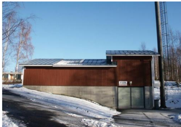
Figure 1. District heating plant in Tuupovaara
